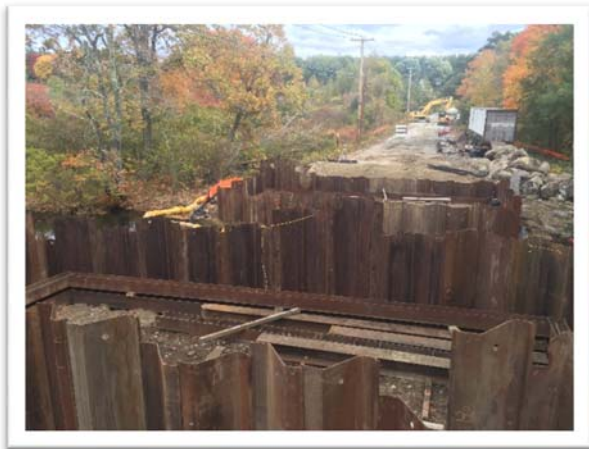
Cofferdam Installation at New West Abutment Location Looking East
