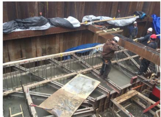
Placing West Abutment Footing Looking East
