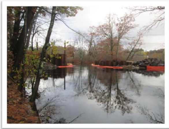
High Water Levels at the Project Site Looking Upstream
