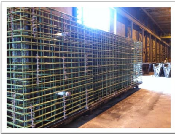
Reinforcing Cage for Precast Bridge Element
