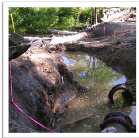
Waterline Excavation Inundated from Heavy Rains
