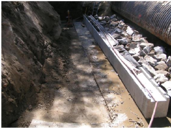
Completed East Footing with Filter Fabric & Rip-Rap
