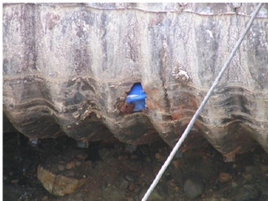
Typical Hole in Existing Culvert
