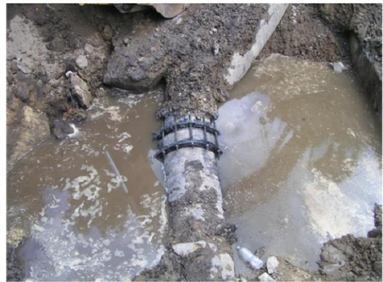
Mechanical Joint Restraint at a lower fitting
