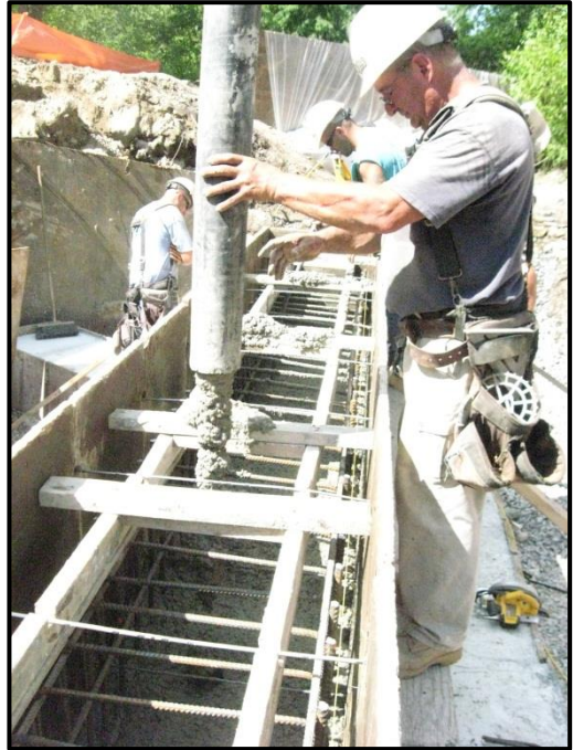
Placement of concrete for one of the stem walls.
