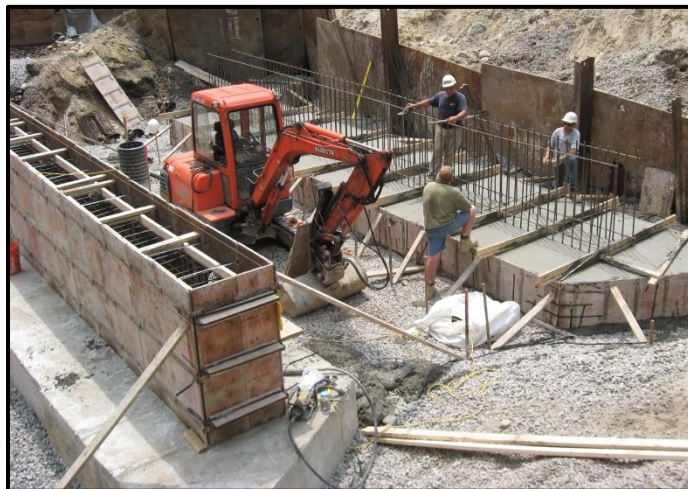
Finishing the freshly placed concrete for the west footing.
