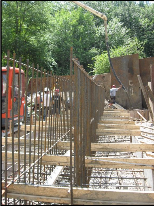
Reinforcing in place for the east footing and stem wall.
