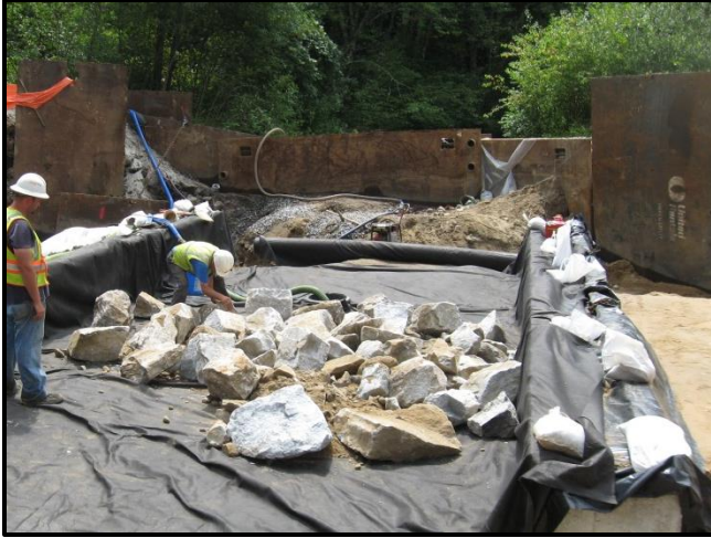
Stone being placed in the new streambed.
