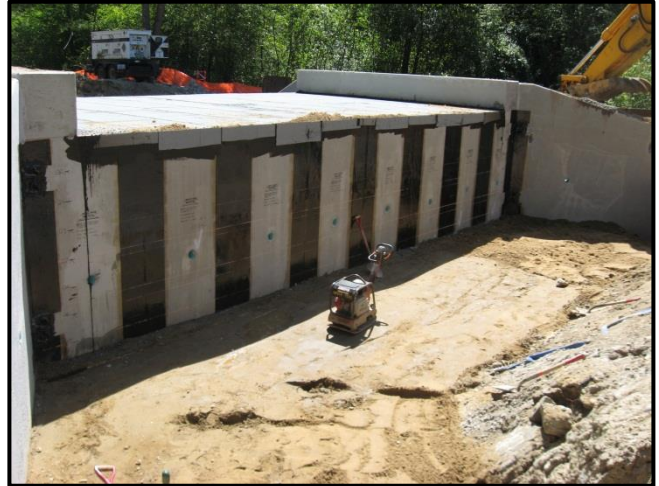
Waterproofing in place on the precast sections and backfilling operations taking place around the structure.
