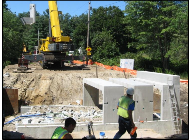
Placement of the precast Rigid Frame Box and wingwall sections.
