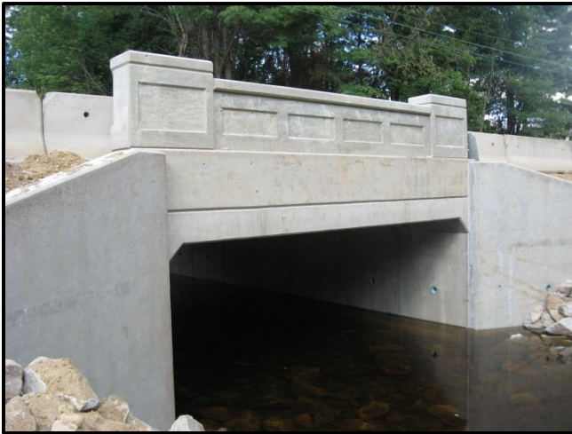
The upstream side of the new culvert with the bridge rail installed.
