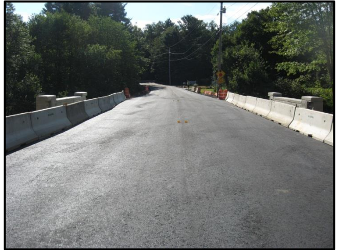
The roadway after placement of the first layer of asphalt.
