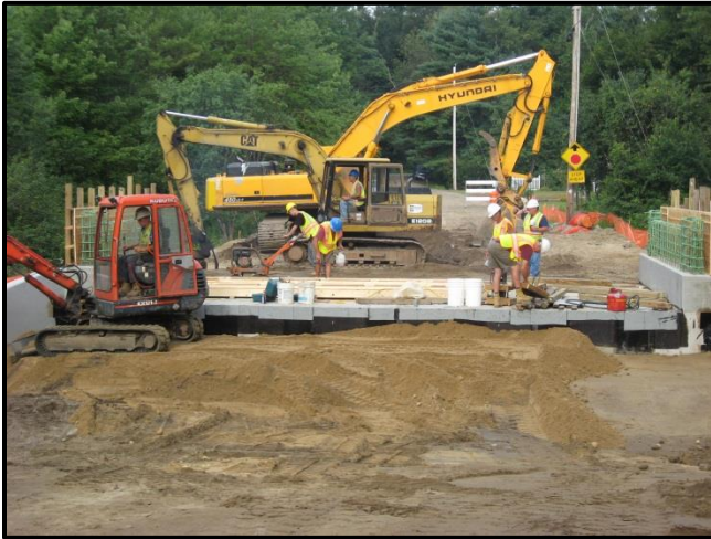
Backfilling operations and preparation for placing the bridge rail concrete.
