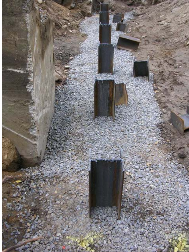
Steel pile cut-offs
