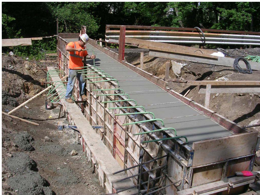
Pouring concrete for west abutment
