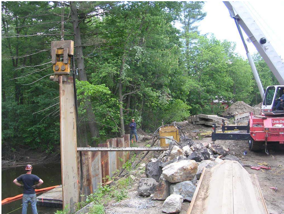
Driving steel sheets for retaining wall construction
