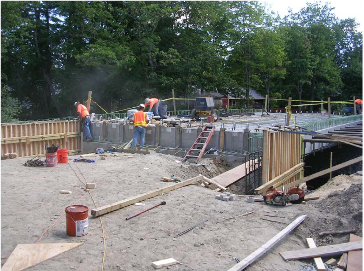
View of box beams and wingwall forms
