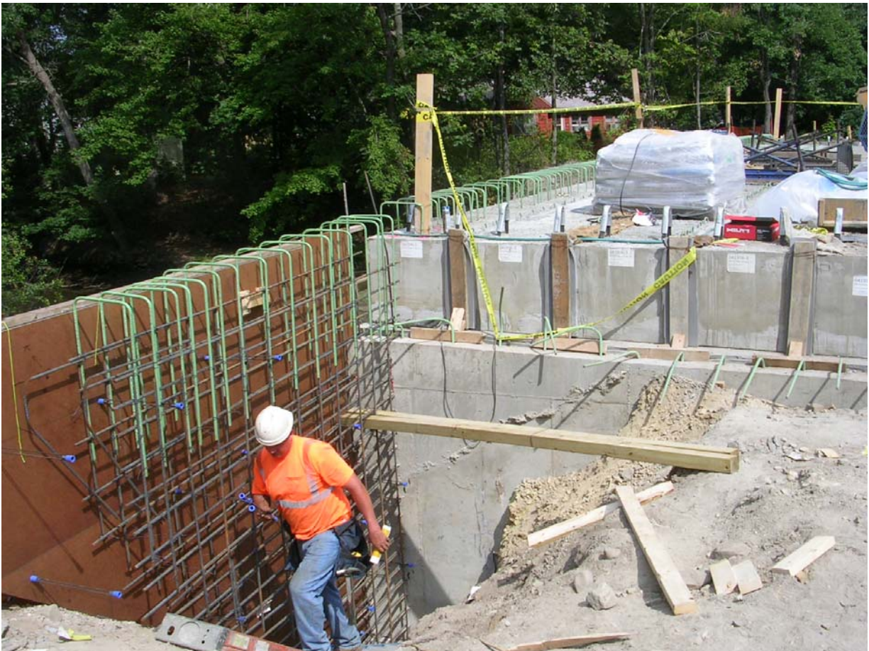
Installing rebar in wingwall
