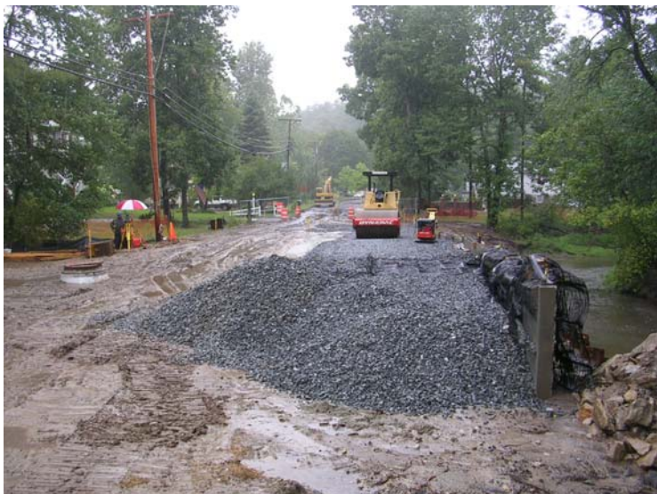
Backfilling at retaining wall
