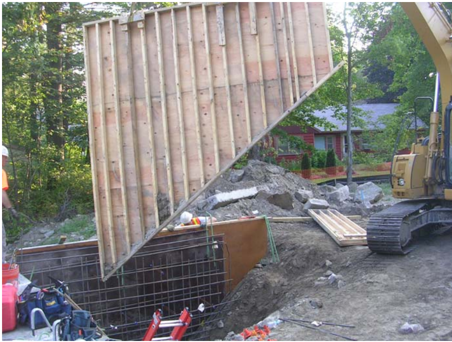
Installing forms for wingwall
