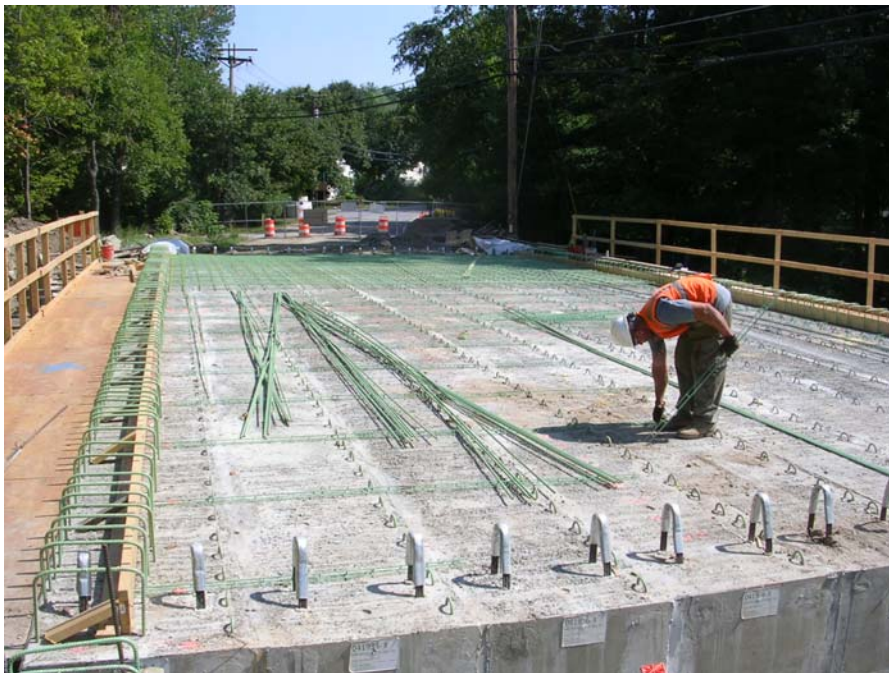
Placing re-steel on bridge deck
