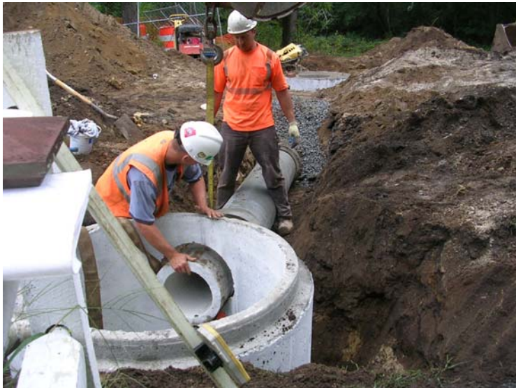
Installing concrete pipe on west approach
