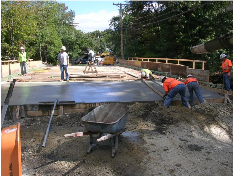
Finishing concrete approach slab
