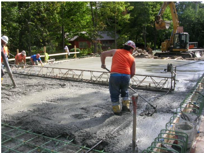
Pouring concrete bridge deck
