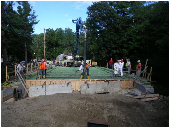
Pouring concrete bridge deck
