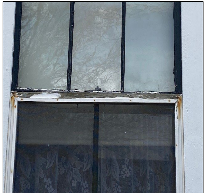
PHOTO – North Elevation, Window on the first floor, north elevation, with rusted screen installed over the lower sash.
