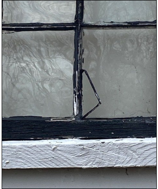
PHOTO 5 – East Elevation, 9/9 double-hung window on the first floor of the east elevation. These may be the oldest surviving windows in the building, potentially dating to the eighteenth century.
