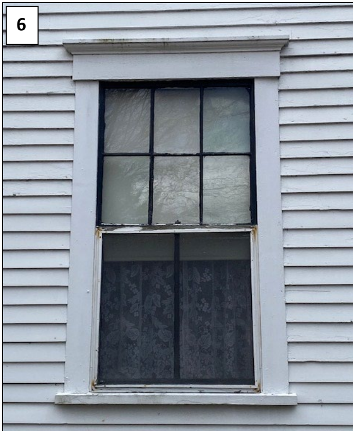
PHOTO – North Elevation, Window on the first floor, north elevation, with rusted screen installed over the lower sash.
