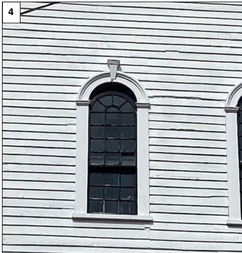
PHOTO 4 - South elevation, paired arched windows and lunette within the gable are twentieth century additions. Glazing putty on each window is visibly lifting or missing.
