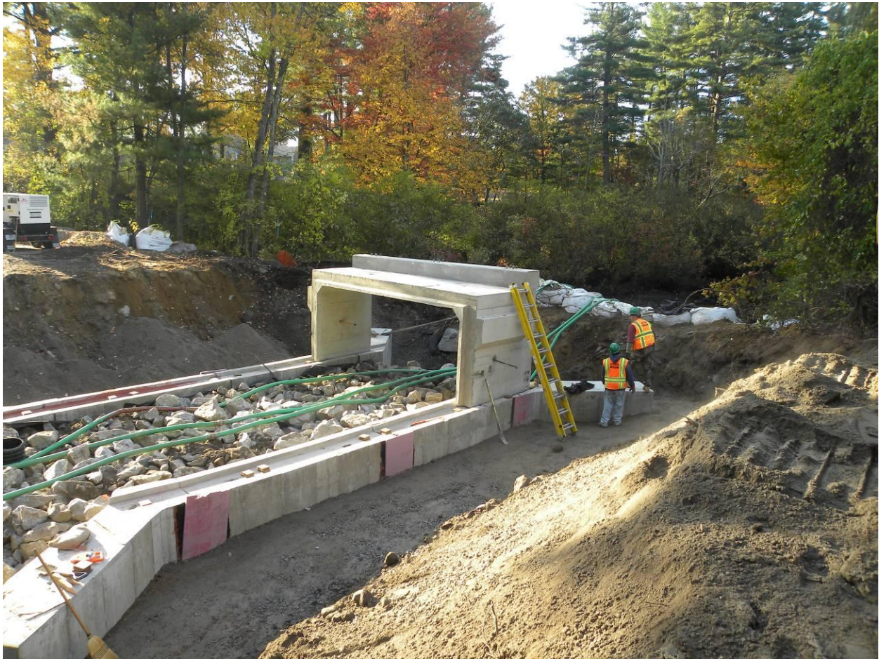
Pre-cast footings and first box section in place.
