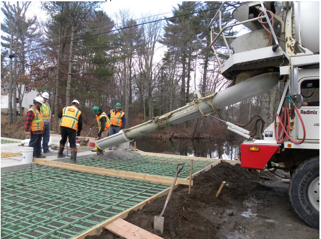
Placement of QA/QC Approach Slabs to bridge.
