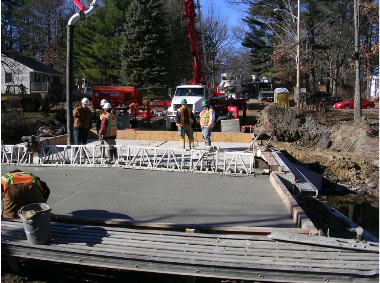
Placement of variable thickness deck overlay.
