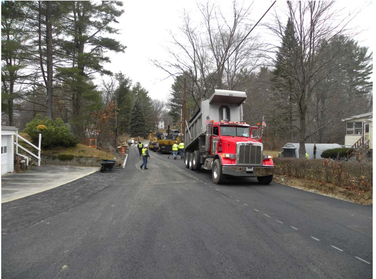
Placement of final pavement over base pavement.
