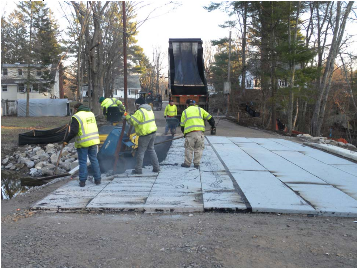
Placement (by hand) of bridge base pavement over membraned bridge deck.
