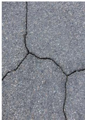
Block Cracking
