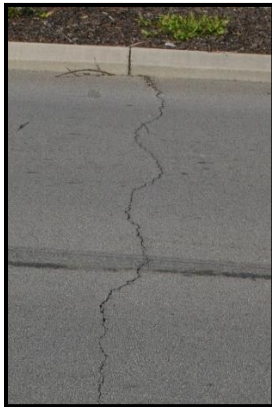
Transverse & Reflective Cracking
