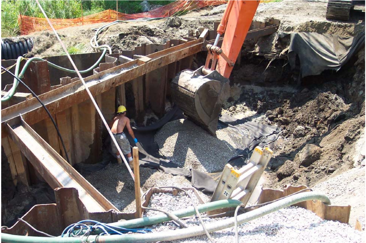
Installation of stone and fabric
