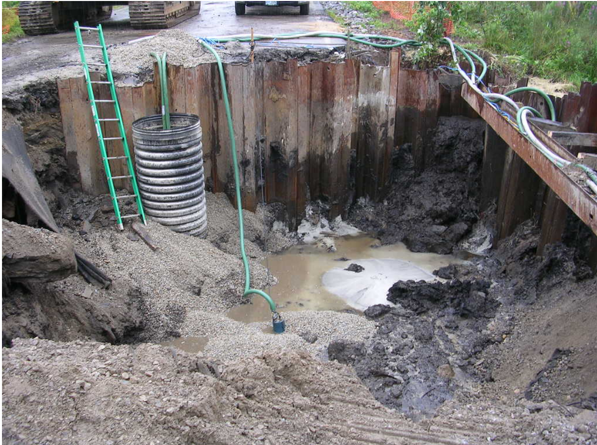
Excavation inside cofferdam
