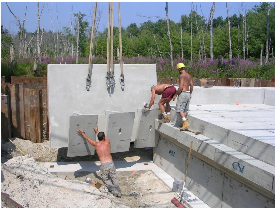
Backfilling around the structure was performed, barrier membrane was placed and preparation for placement of approach slab concrete is underway.
