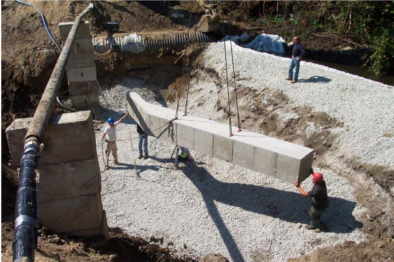
Upstream wing wall footing
