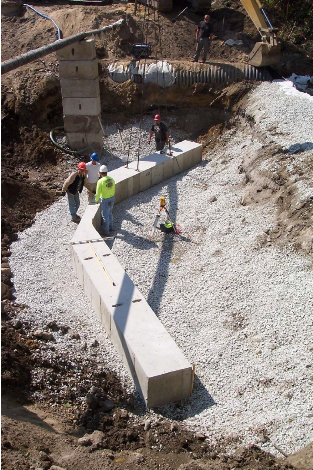
Upstream wing wall footing
