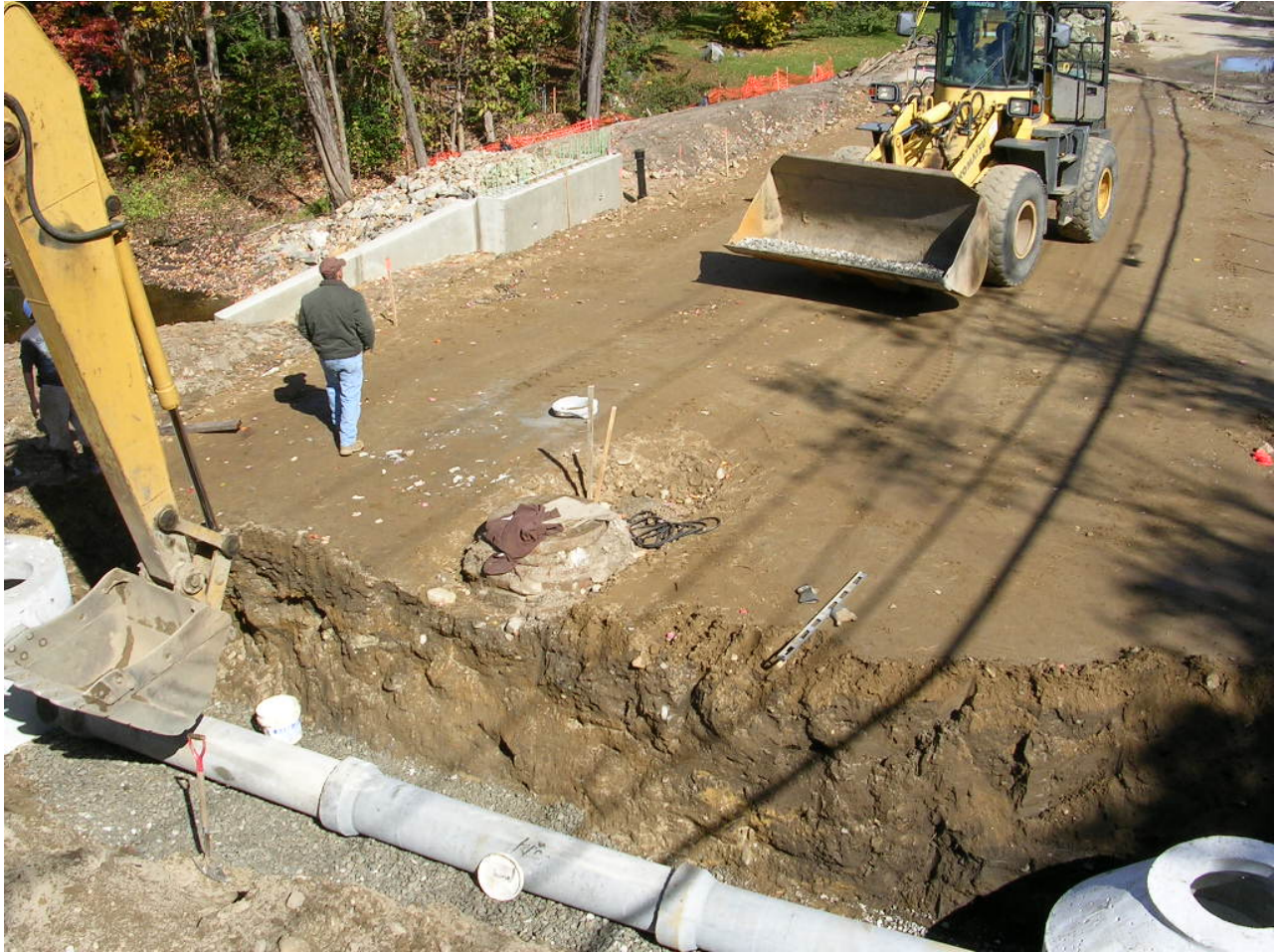
Installing storm drainage
