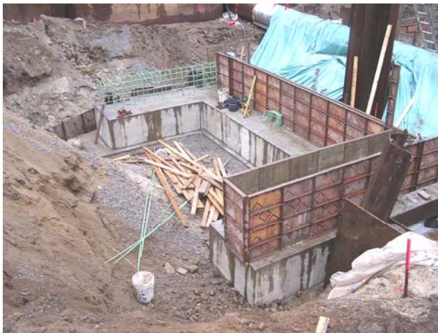
West Pedestal Wall Form work and reinforcing steel (above left) and concrete pour (above right)
