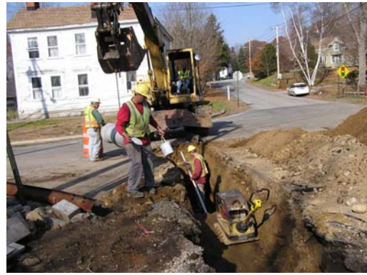
Installation of catch basin and pipe at intersection (above and left)
