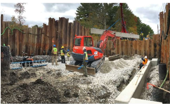
Installing Foundation Footings
