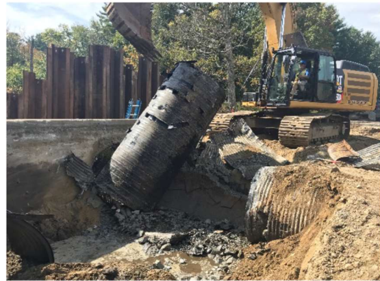
Removing the Existing Culverts
