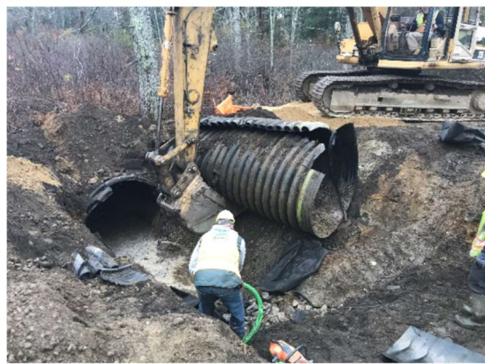
Removal of Water Diversion Culvert
