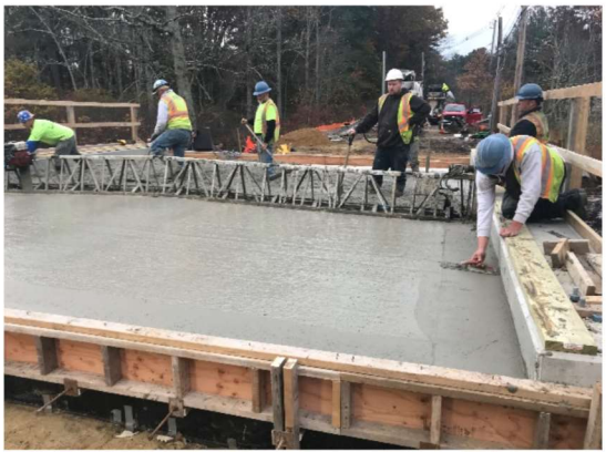
Placement of the Concrete Deck
