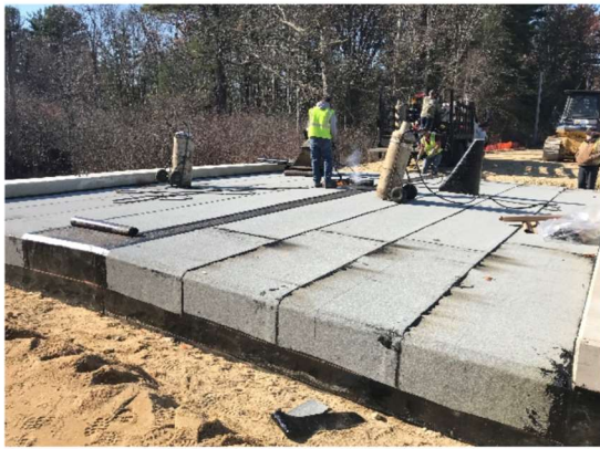
Installation of Deck Waterproofing Membrane
