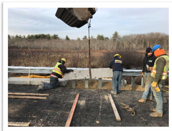
Installation of Granite Curbing
