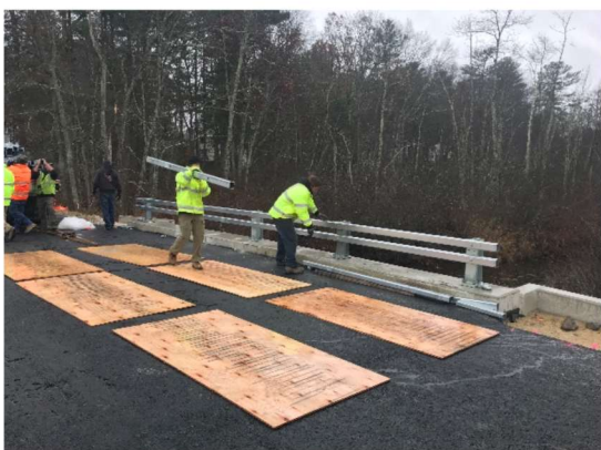
Installation of Bridge Rail
