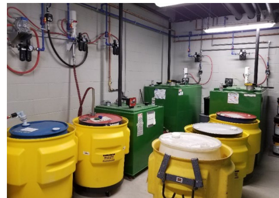
Example of maintenance bays & fluid containment
