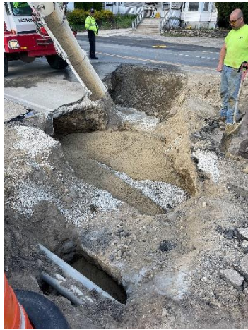
Pouring flowable fill to reinforce undermined duct banks during drainage installation
