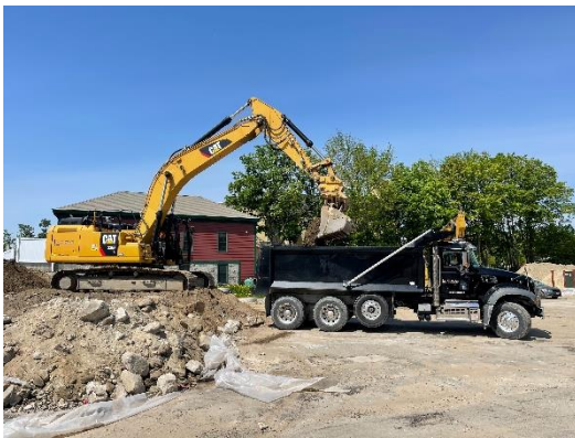
Contractor loading petroleum contaminated soil for disposal off-site.
