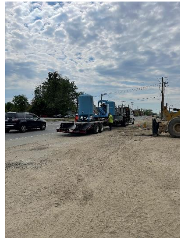
Delivery of the carbon filter water treatment system. This system was used to filter contaminated groundwater.
