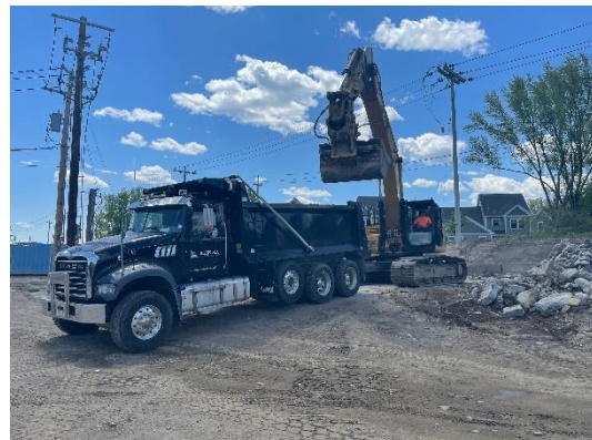
Contractor loading concrete from old drainage infrastructure for disposal off-site.
