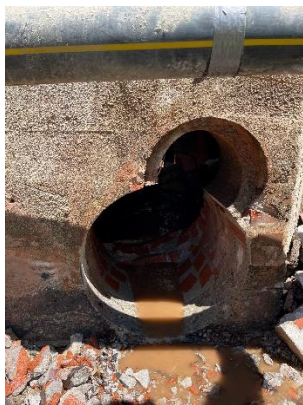
Coring of a drainage structure at Dunkin Donuts to accommodate a larger crossing pipe.
