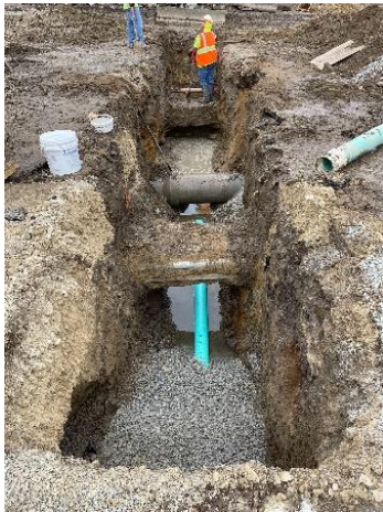
Extension of an existing sewer service at 6 South Broadway
