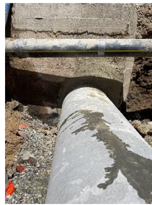
Finished parging of the outside of a drainage structure at Dunkin Donuts to make a watertight seal to the drain pipe.
