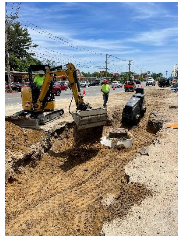
Installation of a new catch basin for the future widening of South Broadway.
