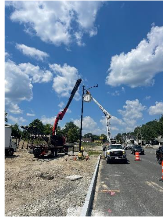
Subcontractor installing new decorative light poles
