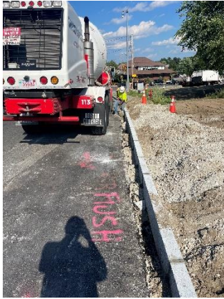
Contractor setting curbing in concrete on Main Street
