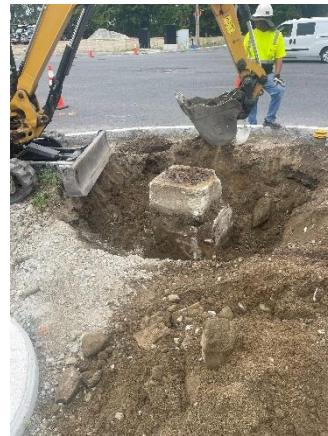
Concrete light pole base being removed to allow for the installation of new sidewalk at the intersection.
