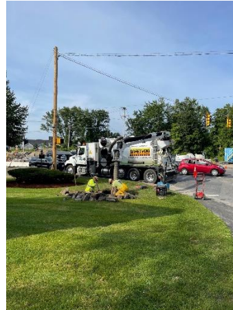
Large vacuum truck excavates for new traffic signal mast arm foundation adjacent to Salem Co-operative Bank.
