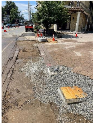
New foundation installed for crosswalk pushbutton at the Rail Trail crossing.
