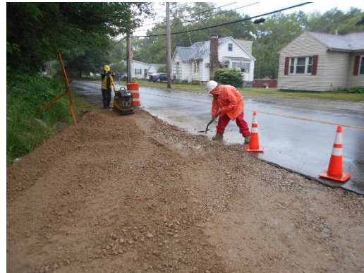
Grading/compacting at North Main Street
