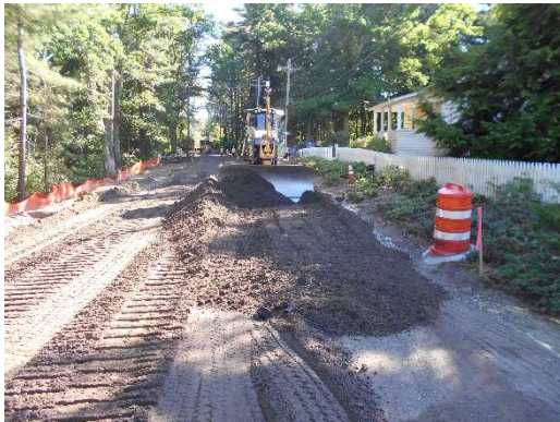
Spreading gravel
