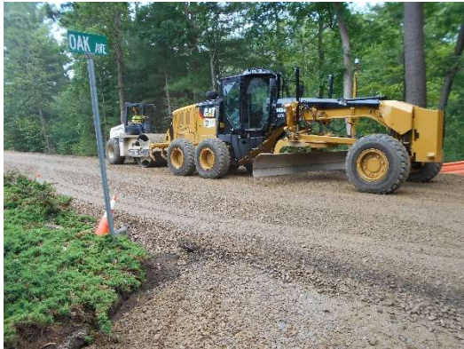
Grading and compacting roadway gravel.
