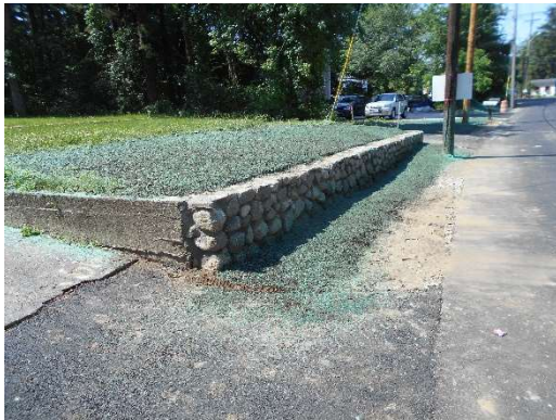
Relocated retaining wall.
