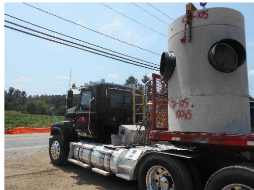
Drainage structure delivery.
