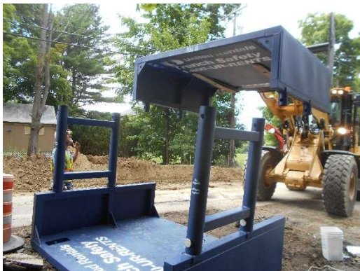
Assembling new trench box for deep catch basin installations.
