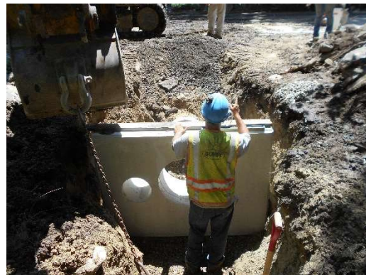
Installing a headwall
