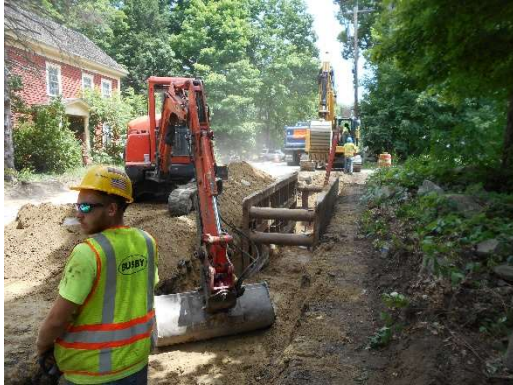
Using trench box for deeper pipe installations.
