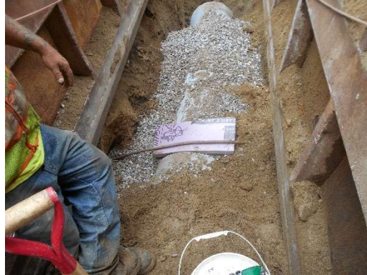
Passing beneath a water service pipe.
