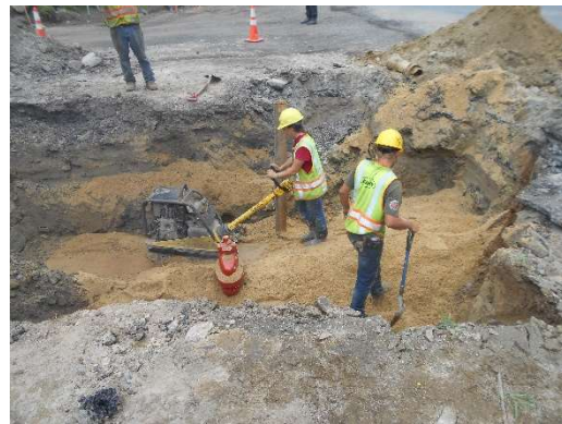
Backfilling in lifts.
