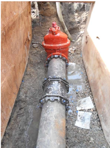
Replacing 12" valve on water main.
