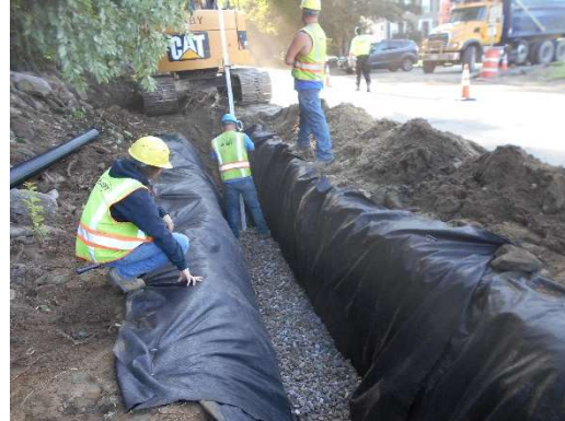
Installing underdrain pipe.
