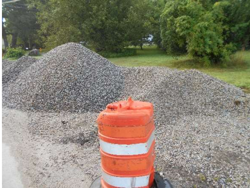
Stone for pipe bedding.
