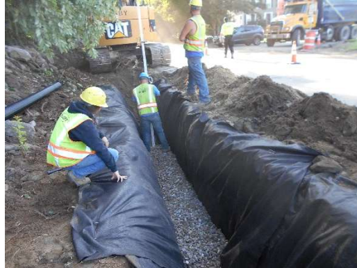
Installing underdrain pipe.
