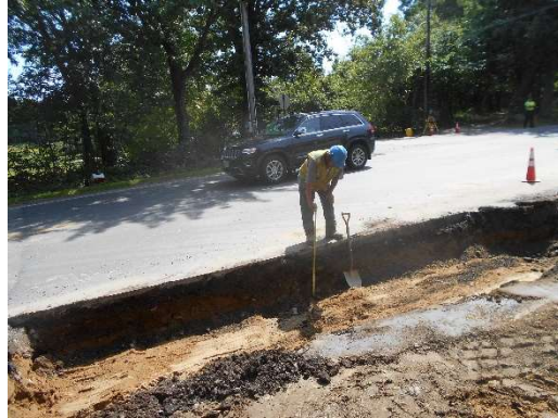
Excavate poor soil and install gravel.
