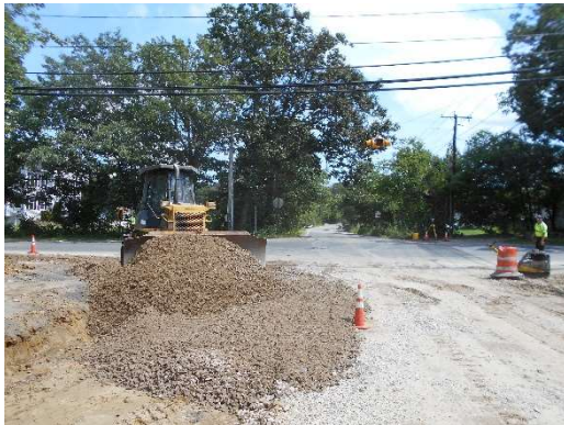
Spreading the gravel.
