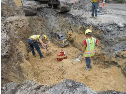
Backfilling a water gate valve.
