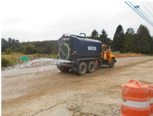
Two benefits to watering gravel: dust control and better soil compaction.
