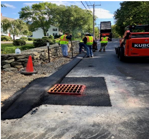
10/01/18-Install Bit Curb - Zion Hill Rd.
