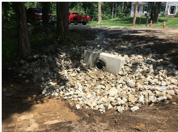
7/29/18 – Headwall Installation on Captains Rd
