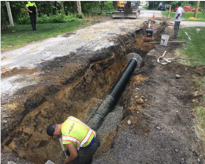
7/12/18 – Drainage installment on Captains Rd
