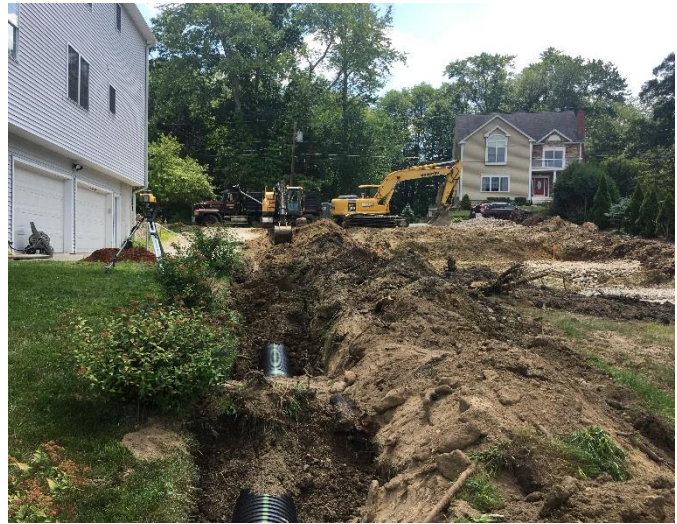
7/13/18– Drainage installment down to Captains Pond
