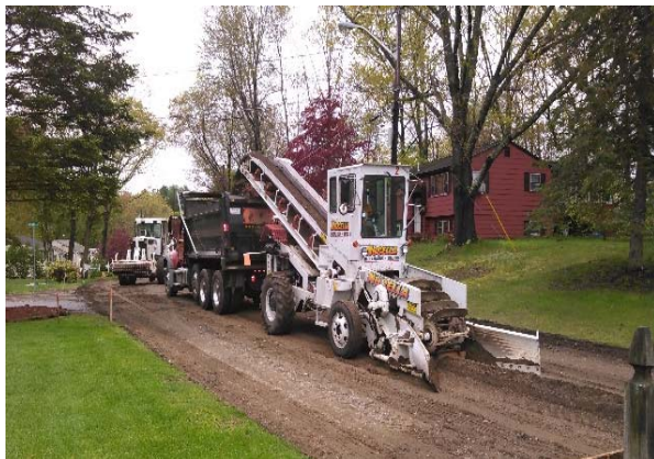
5/15/17 – Reclaim Operation on Bradford Drive near Grove Ave.
