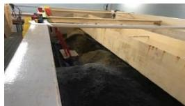
some of the braces holding the underdrains in place have shifted or become bowed over time. To address this, we will need to remove all the filter media, complete the required repairs, and replace the filter media. This work is expected to take approximately three weeks due to product availability.
