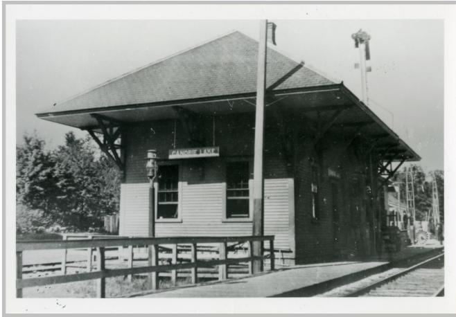
Canobie Lake Train Station: The first railroad station constructed near this location was named Policy Pond after the adjacent pond, now known as Canobie Lake. In 1885 the station was reconstructed to meet the growing popularity of the area by offering passenger service along with freight. The new station was named Canobie Lake by the Railroad Commissioners in honor of Canonbie, a small village in Scotland, in recognition of local heritage at the time. The distinguished name was chosen to promote the area as a destination for vacationers and tourists, subsequently Policy Pond itself was renamed Canobie Lake.
