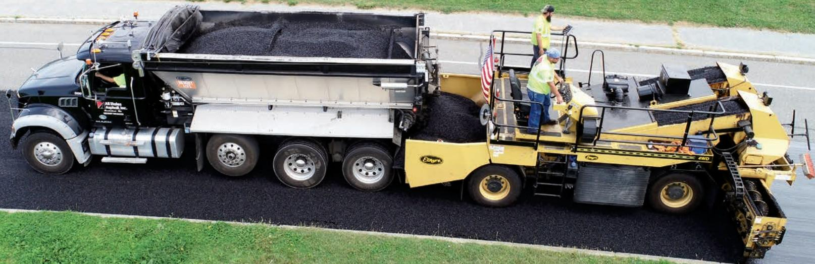
SAM construction differs in that binder sprayed on the existing pavement is liquid asphalt rubber, and the stone has been pre-coated with a performance grade liquid asphalt before it is spread on the road and rolled.
