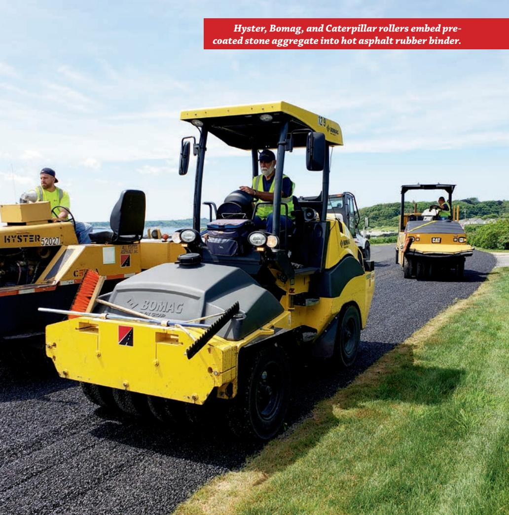
*Hyster, Bomag, and Caterpillar rollers embed pre-coated stone aggregate into hot asphalt rubber binder.*
