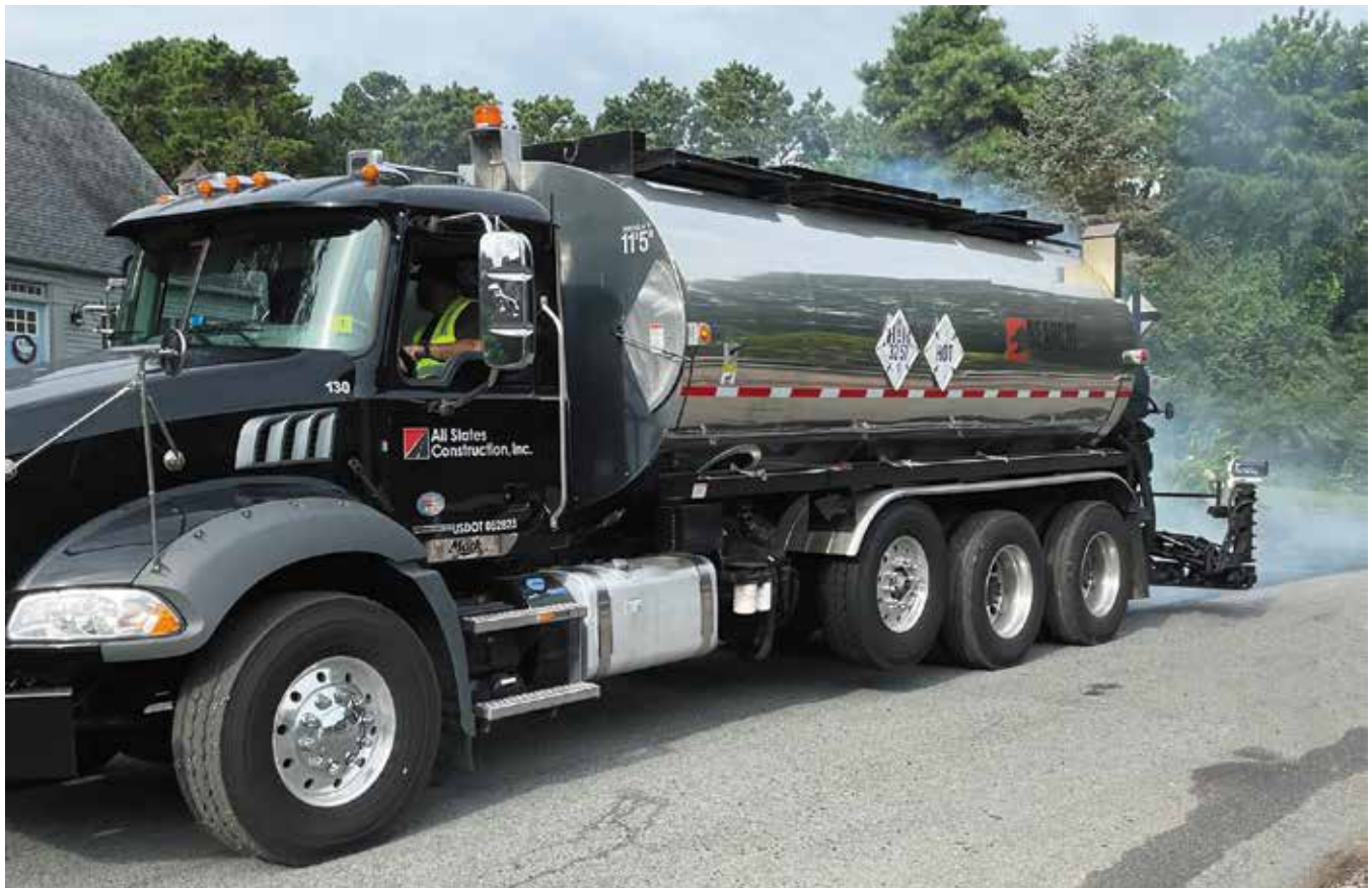
In Yarmouth, All States Construction places hot spray crumb-rubber modified asphalt seal, to be followed immediately by chip spreader
