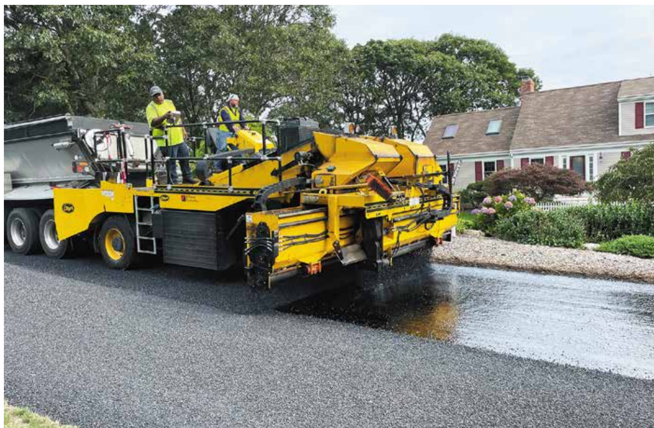
Application of heated and pre-treated 7/16-in. aggregate as part of the asphalt-rubber chip seal process in Yarmouth, Mass.
