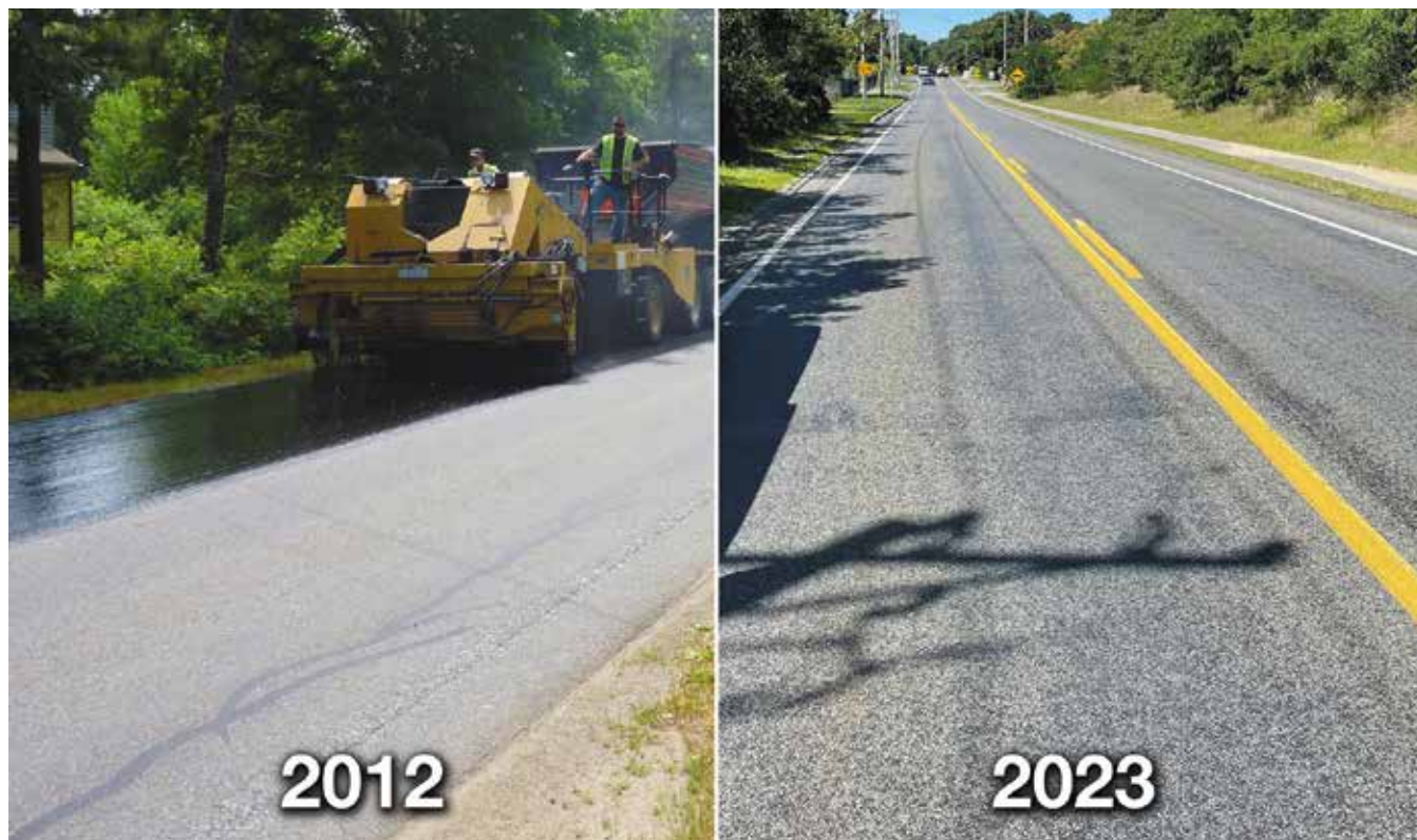
Camp Street in Yarmouth during application of the asphalt rubber chip seal in 2012 (left) and after 11 years of in-place performance
