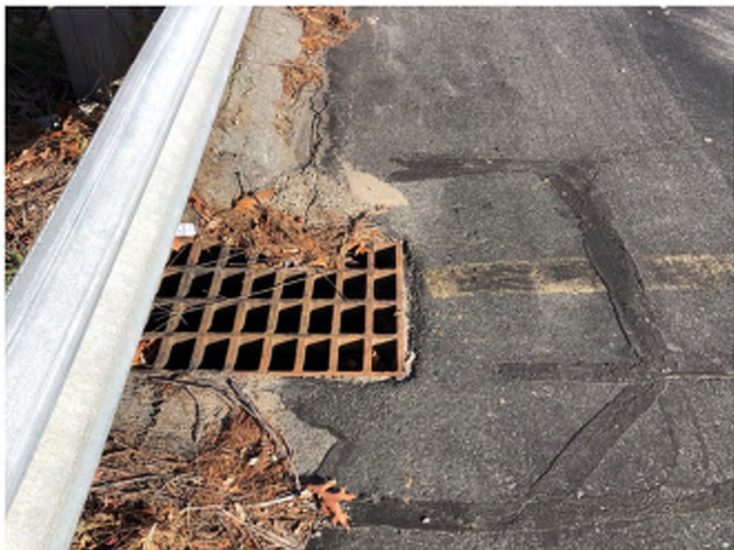
Close up of catch basin on western edge of Eastbound NH111.
