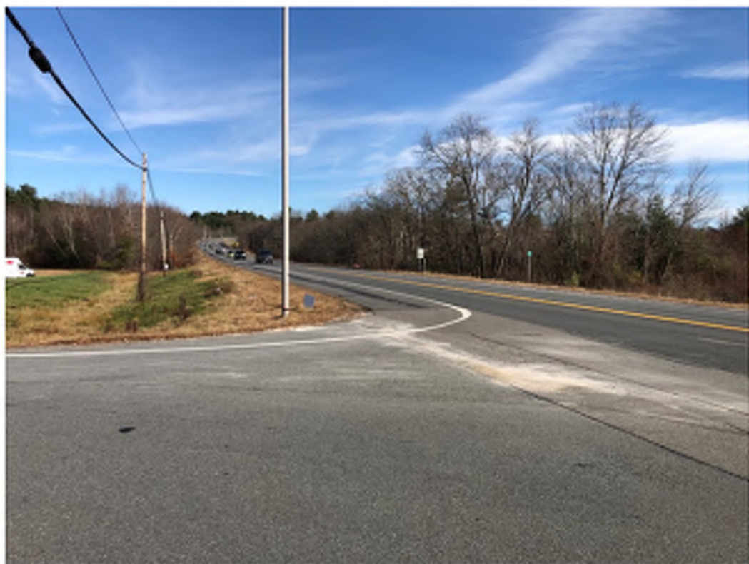
View toward eastbound NH111 from Ermer Road, pointed NE. Note the proximity of the light pole to the edge of pavement as well as the slope leading away from the roadway.
