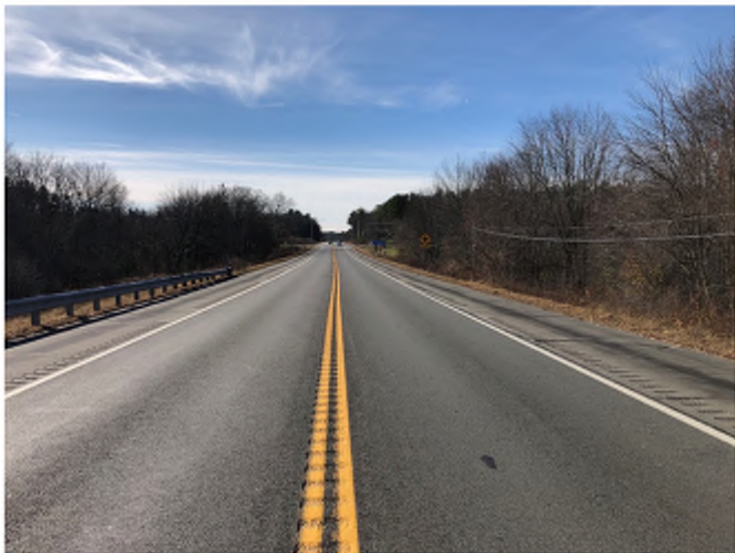
View facing SW toward the Ermer Road-NH111 intersection from NH111 east of intersection. Note centerline and edgeline rumble strips.
