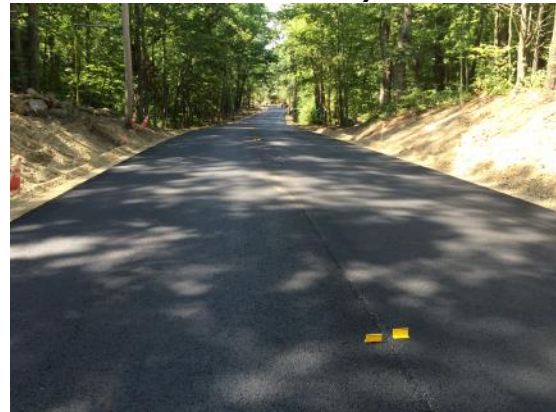
Completed Binder Course Pavement near 68 Haverhill Road
