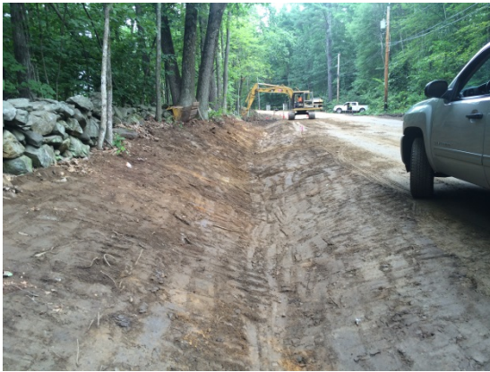
Swale construction (Opposite from 76 Haverhill Road)
