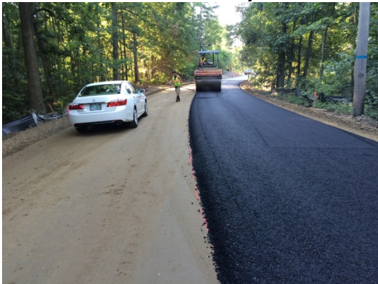
Paving Binder Course (Near 62 Haverhill Road)
