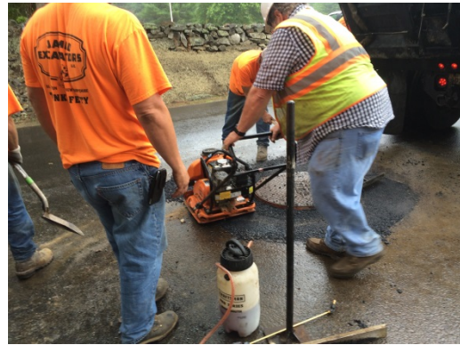
Drainage Structure Adjustment near 43 Haverhill Road
