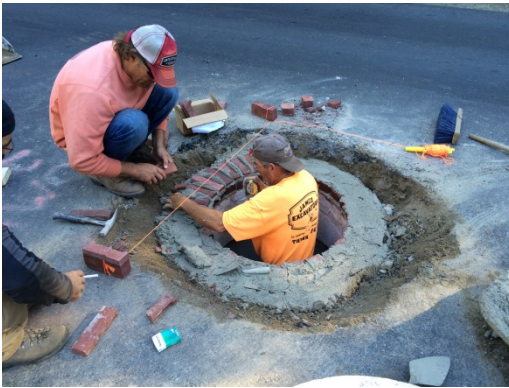
Drainage Structure Adjustment near 41 Haverhill Road
