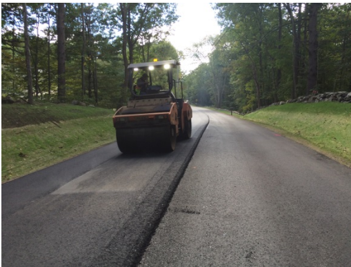
Top Course Pavement Installation
