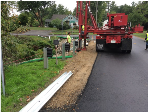
Guardrail Installation near Old Farm Road
