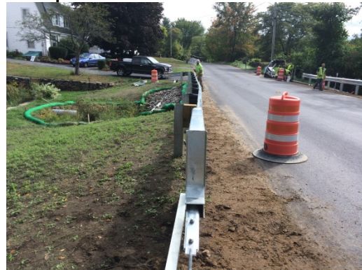
Guardrail Installation near Old Farm Road
